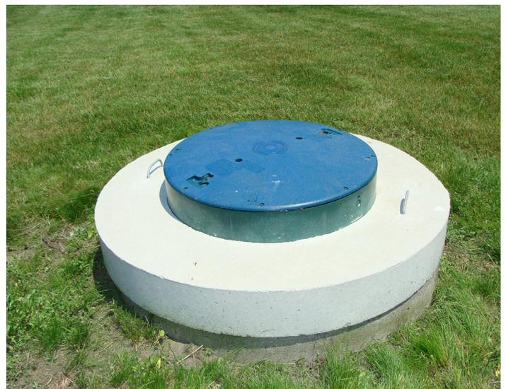
*A dug well with an upgraded sturdy lid (that is properly vented and vermin proof) reduces the amount of contamination that can enter the well. Older wells of this type may have been constructed with stones, bricks, or other materials. The coloured portion of this well lid allows for observation of the well without having to removing the heavy concrete lid. The concrete lid can be removed if maintenance is required.*
