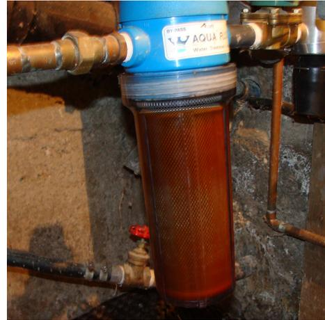
*A water treatment filter. Equipment requires regular inspection and maintenance. This filter needs to be replaced.*
