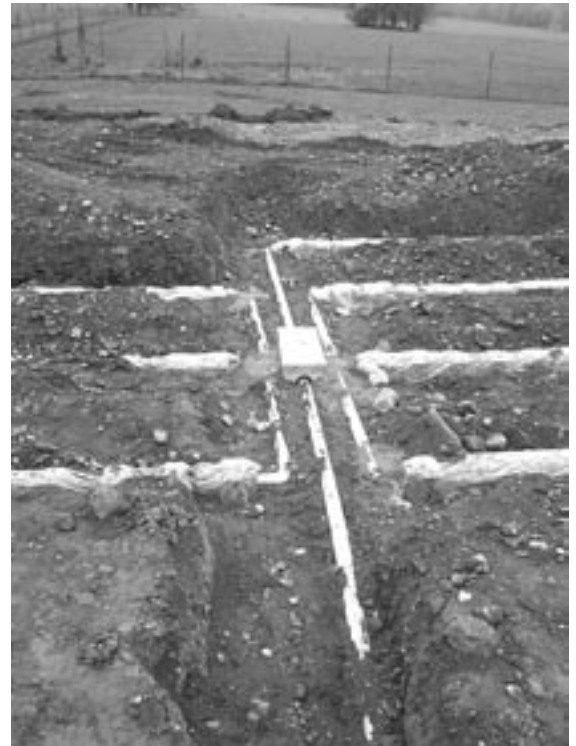
Overview of a new septic bed before being covered
