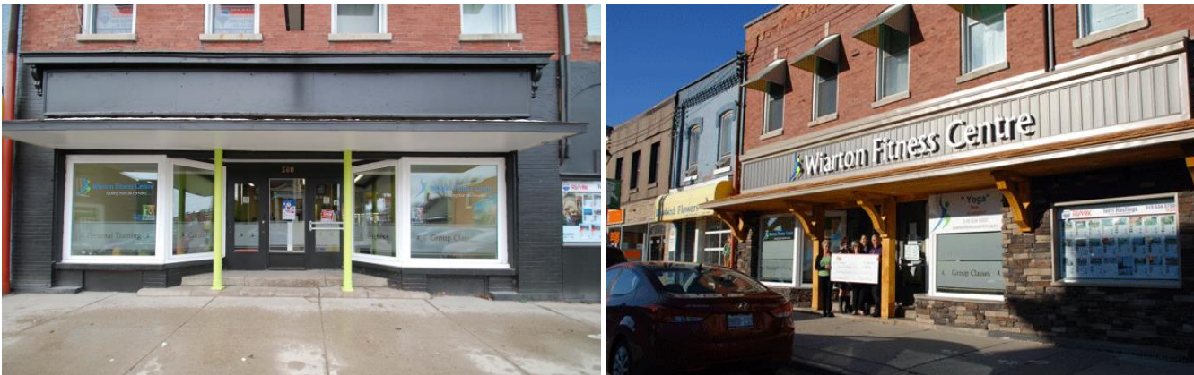
The Warton Fitness Centre, before (left) and after facade improvements funded by the "Spruce the Bruce" program (right).
