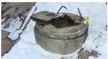
It is important to regularly inspect and maintain your well and test the water. This is a drilled well located in a pit (these are no longer allowed to be constructed). If you have a well located in a pit, you could upgrade it so that the well casing extends at least 40 cm above the ground. NEVER ENTER A PIT.
