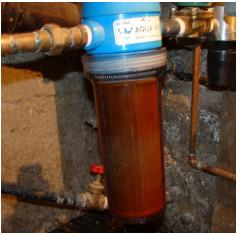
A water treatment filter. Equipment requires regular inspection and maintenance. This filter needs to be replaced.
