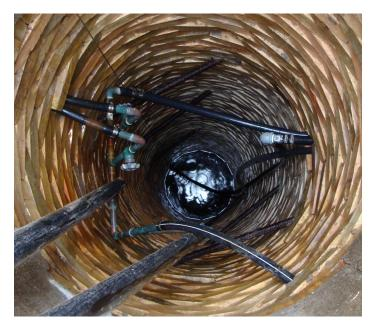
A dug well that is over 100 years old. Moisture seen on the concrete and tile casings indicates that surface water is getting into the well. Ensure that the well is constructed and maintained properly to reduce potential contamination from entering the well.
