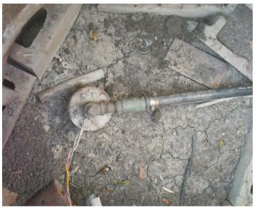
The soil is cracked, evidence that water has entered the well pit (not to be constructed this way anymore) and dried. One way to prevent this from happening is to upgrade the well by installing a pit-less adapter and extending the well casing at least 40 cm above the ground; and ensuring that construction/maintenance is conducted properly. New construction wells cannot be located in well pits. NEVER ENTER A PIT.
