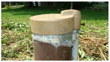
An inadequate well cap may allow pests and other types of contamination to enter into the well, and may not allow for proper ventilation.
