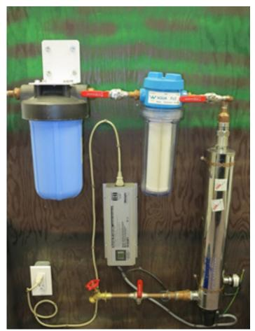
An example of a filter and ultraviolet disinfection system.
