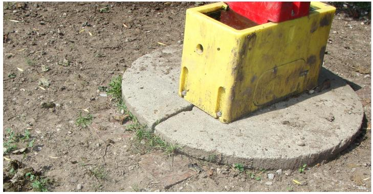
This picture shows the gap in the concrete well cap and its location in relation to the ground and potential sources of contamination.
