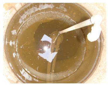
A drilled well located in a well pit (these are not to be newly constructed anymore) can be contaminated when the pit is exposed to surface water (that comes through the casing or through gaps in the cap). These wells can be upgraded to have a pit-less adapter that makes the well more secure and less likely to be contaminated. You can see evidence of water entering the well around the concrete casing joints. New construction wells cannot be located in well pits. NEVER ENTER A PIT.Wells located
