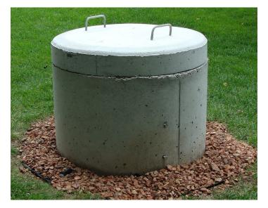
Bored wells with proper casings and sturdy well caps will help to prevent accidental falls into the well and reduce the amount of contamination that can enter the well. As with any type of well, they must be constructed and maintained properly to reduce the risk of contamination and injury.
