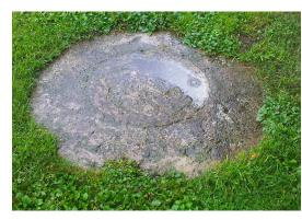
dug well. The well cap is located close to the ground and the well prone to contamination. Know where your well is, how it is constructed and maintained. and how vulnerable it is to contamination.
