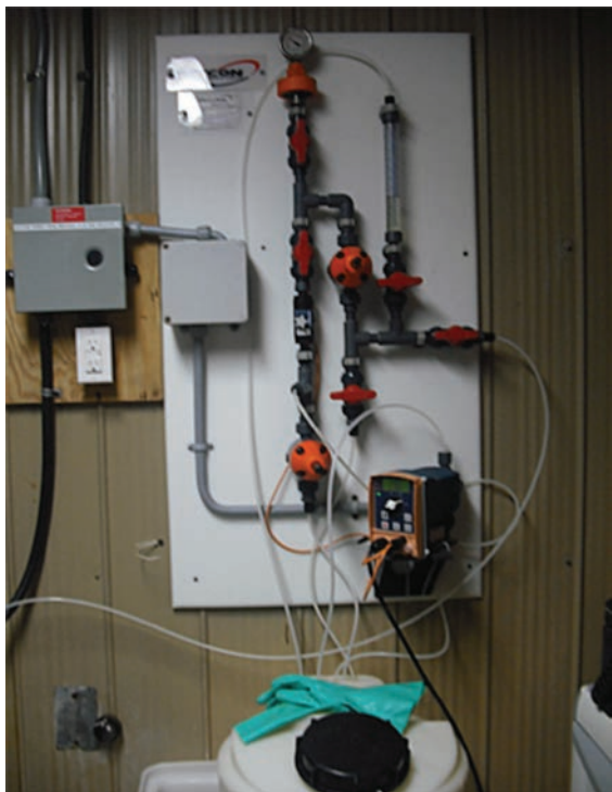
Figure 3: Chlorine Injector
