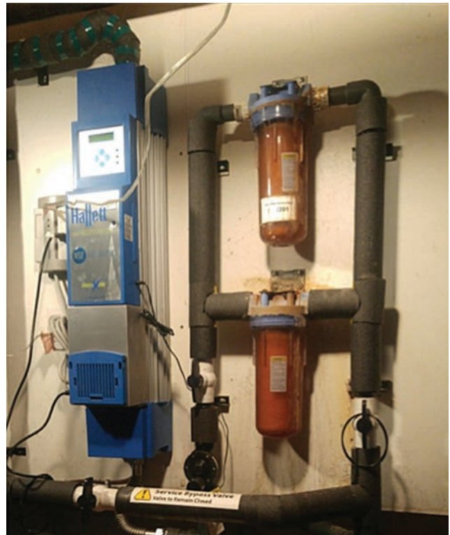
Figure 2: Ultraviolet Light System
